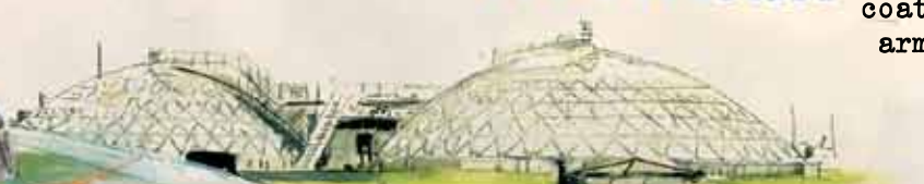
Jackson Pike Sewage Plant's anaerobic digesters
